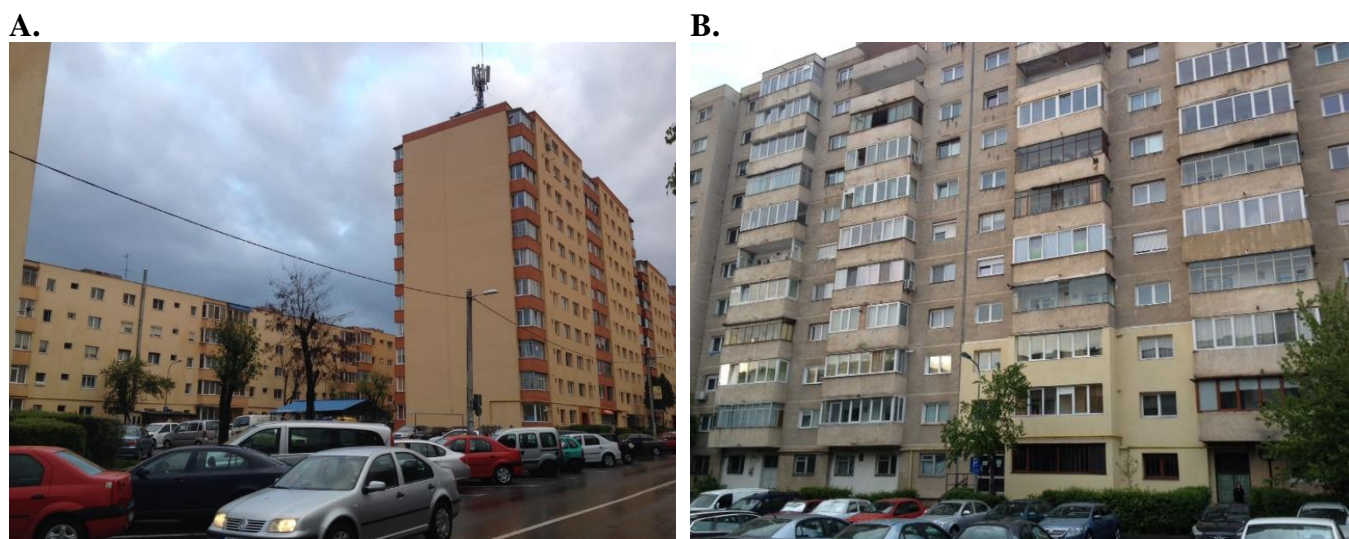
Figure 1: Typical rented social housing in Romania: A. refurbished; B. not refurbished
